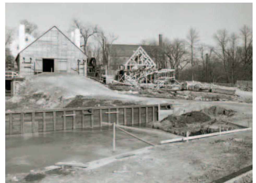
Above: The Iron Works during reconstruction
